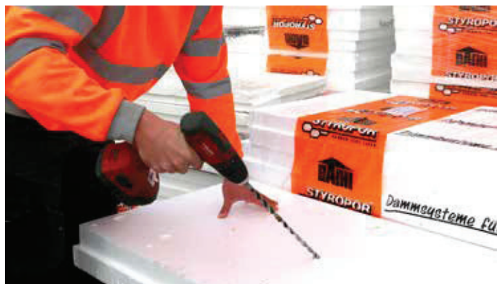
Installation of the ThermoPins made by BT Innovation ... Einbau des ThermoPins von BT innovation ...
