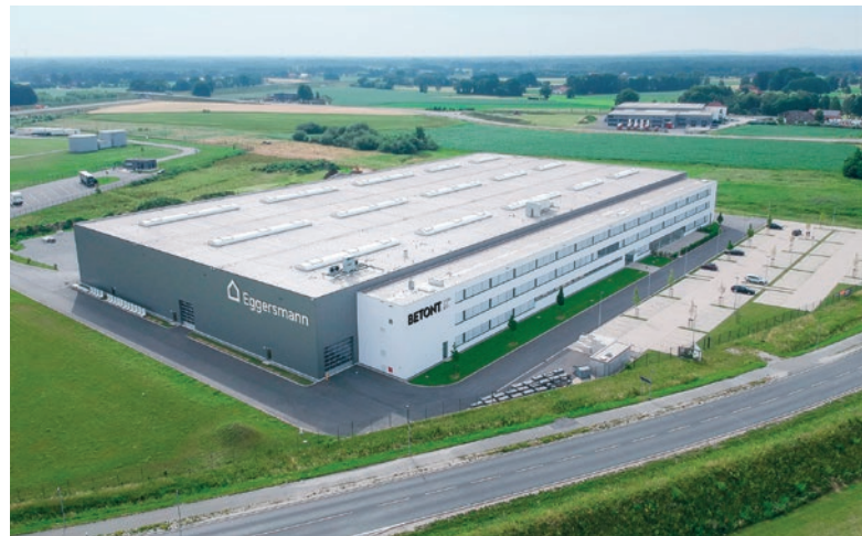
Betont GmbH company building in Halle (Westphalia)
