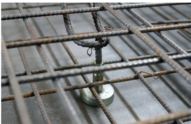
Magnet type GB used as armature mounting
