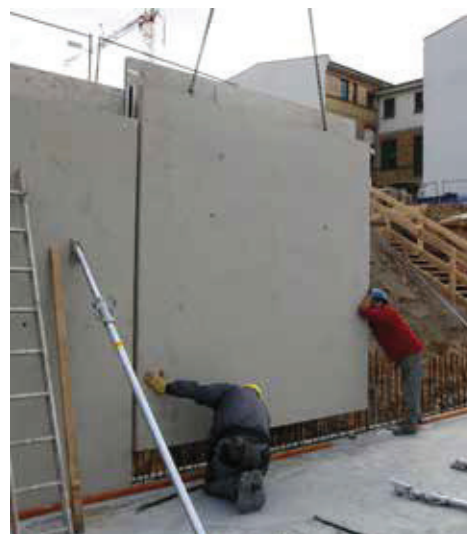
Installation of double wall elements and SynkoElast crack control profiles
