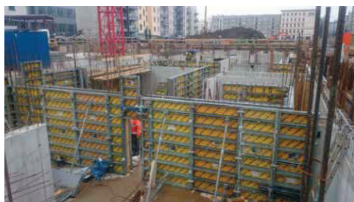
Installation of basement walls as in-situ concrete walls and element walls
