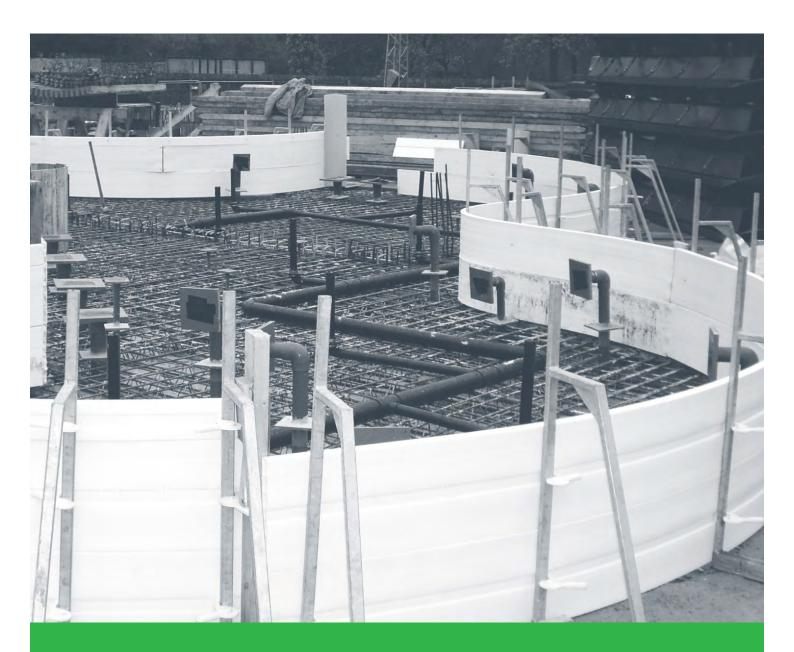
Flexible Formwork for Straight Lines and Concrete Curves
