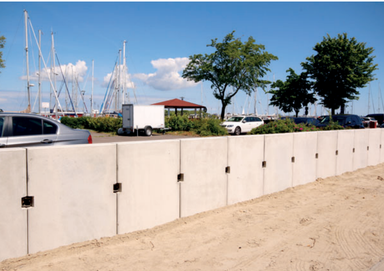
Finished flood protection wall with the BT-Spannschloss in Heiligenhafen
