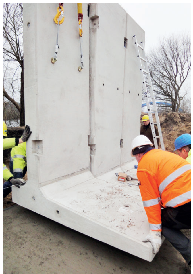
Placement of L-shaped retaining walls in Wittenberge
