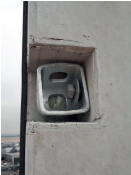
Pre-assembled BT turnbuckle in the recess provided for it
