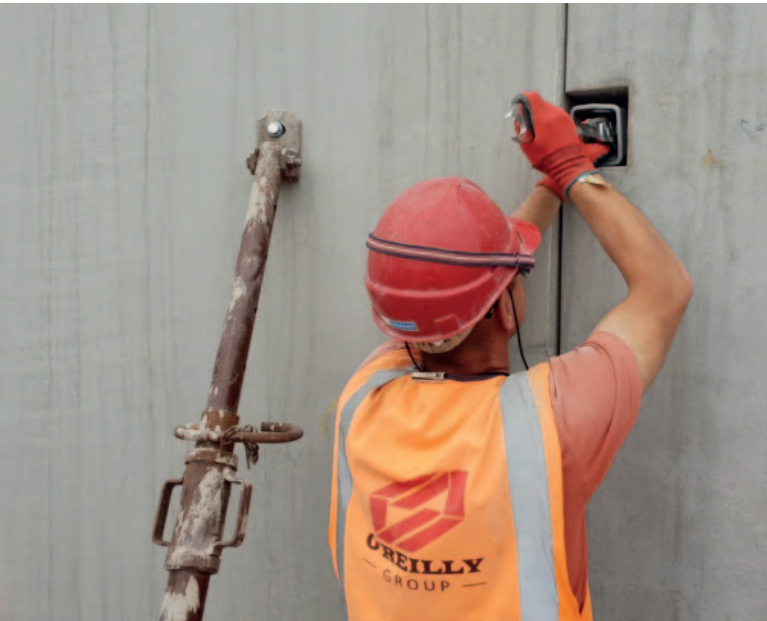
The turnbuckles are tightened in parallel and in a criss-cross pattern using a ring ratchet wrench.
