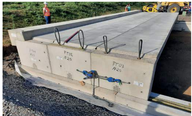
Pre-assembly with chain hoist
