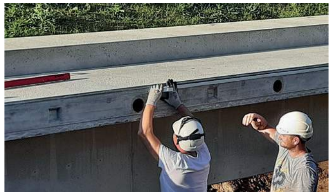
Applying the RubberElast crush joint tape
