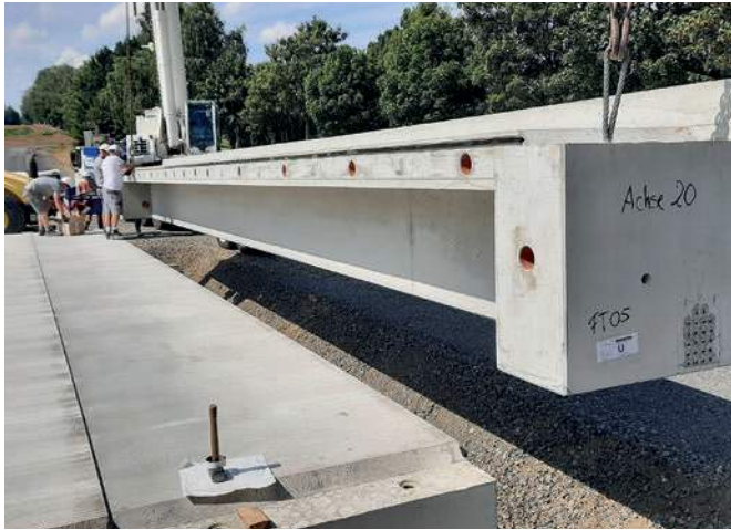
Attaching the last precast element
