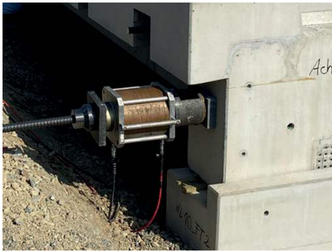
Subsequent cross bracing
