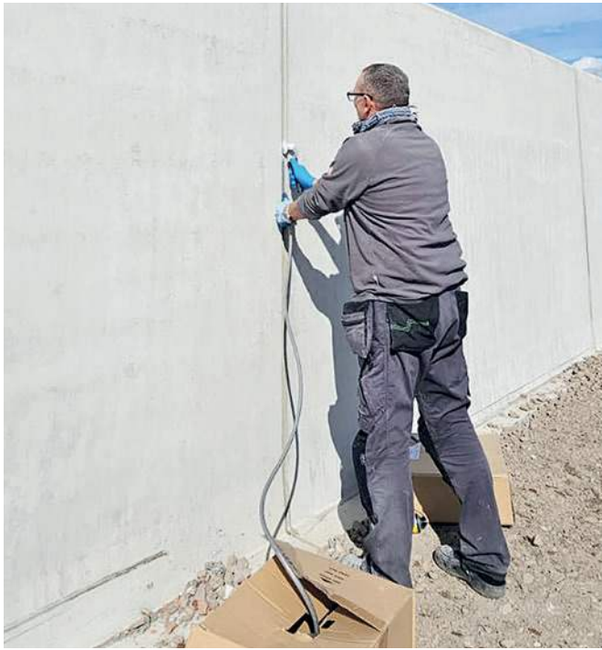
Insert backfill cord
