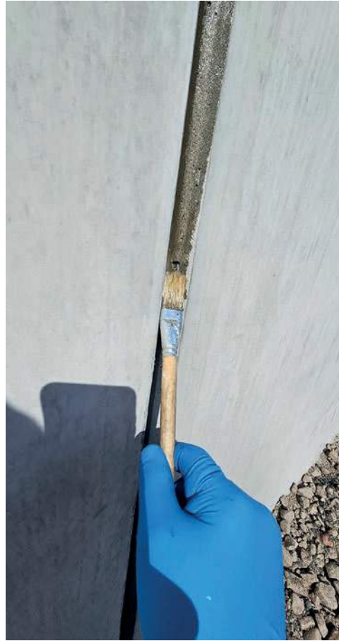
Joint is treated with B(eton) primer
