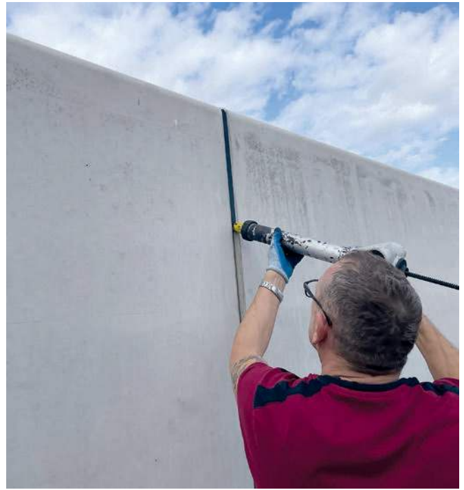
Filling the joint with AgrarElast
