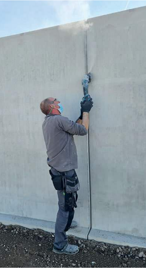
Angular grinding of the concrete joint
