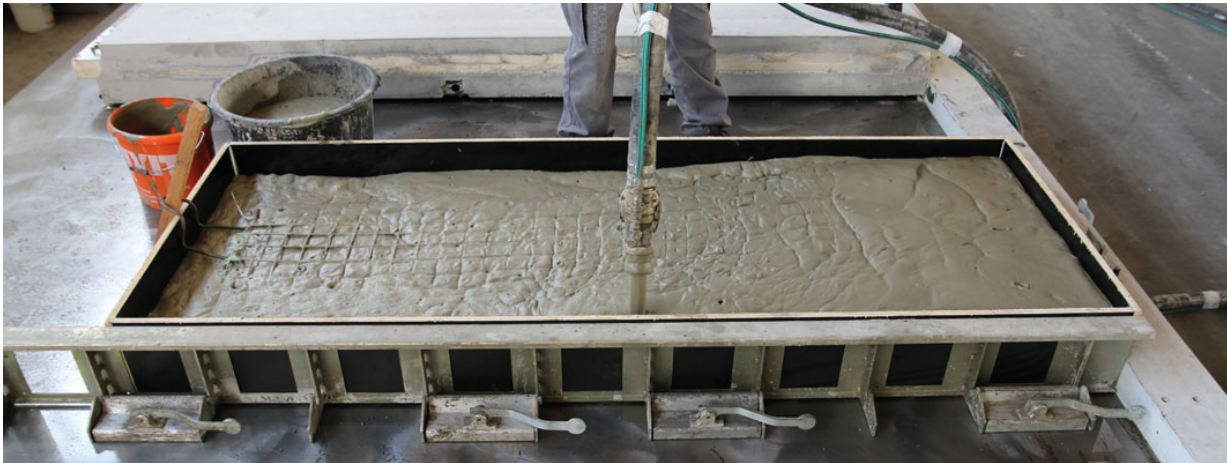
Fig. 3: Horizontal production of a foam concrete wall. The wall had a thickness of 25 cm and was used to determine reference values for the vertical wall.
