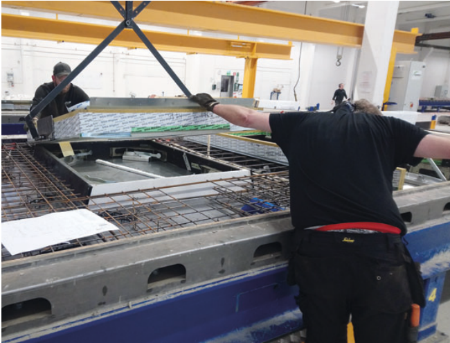
Fig. 6: Window installation in the pallet
