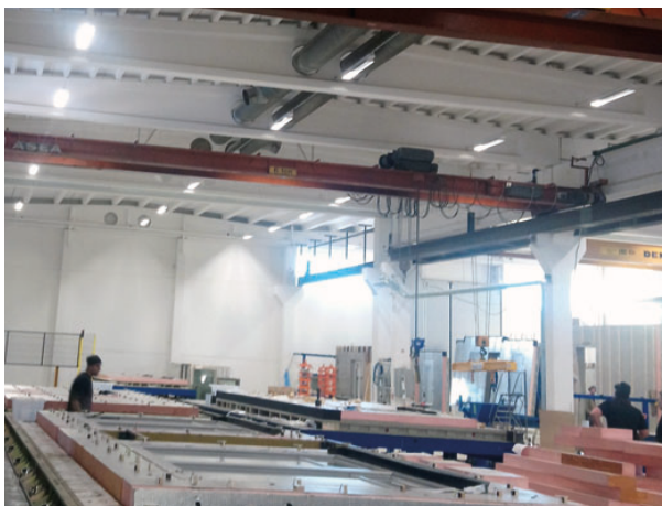
Fig. 8: Installation of the insulation by means of a laser
