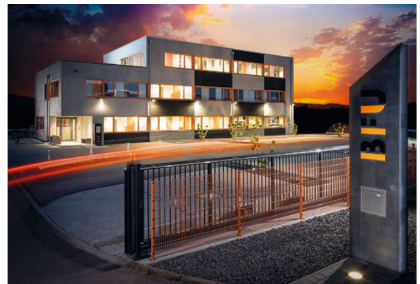
Fig. 2: The BFU headquarters in Schramberg-Waldmössingen was built in 2013 - of course using precast concrete elements from the company's own production.
