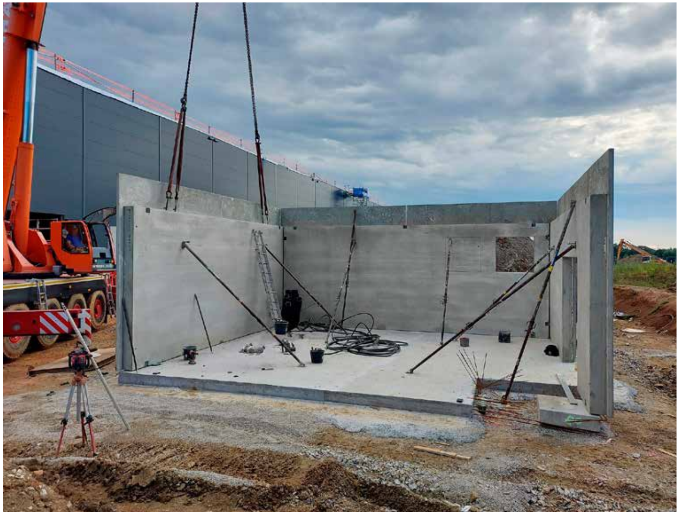
View onto the sprinkler control center after the assembly of three wall panels on the in-situ concrete ground slab
