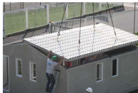
6. Assembling the gabled roof
