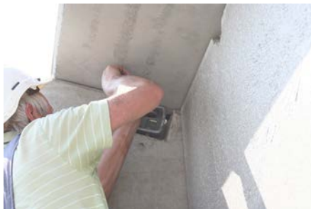
3. Joining system with BT-Spanschloss®
