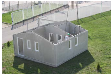
2. Putting the wall components in
