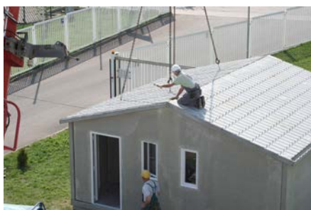
7. Assembling the other side of the roof
