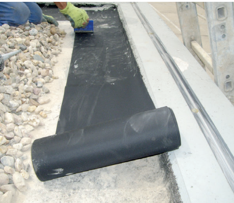
Roof waterproofing with the ProElast® system
