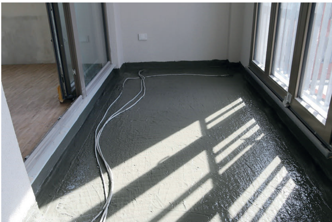
Balcony water- proofing with FlächenElast® system
